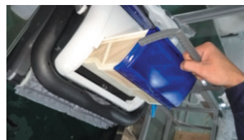
2. Lift the filter tray
